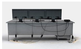
Conventional solution Messy cabling
